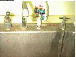
Turn on the water and allow it to run in a steady stream for 5 to 6 minutes. This will ensure that the line is flushed sufficiently to get a representative sample of the water from the distribution system. Additional time might be needed if the water tap is located a long distant from the main distribution line.
