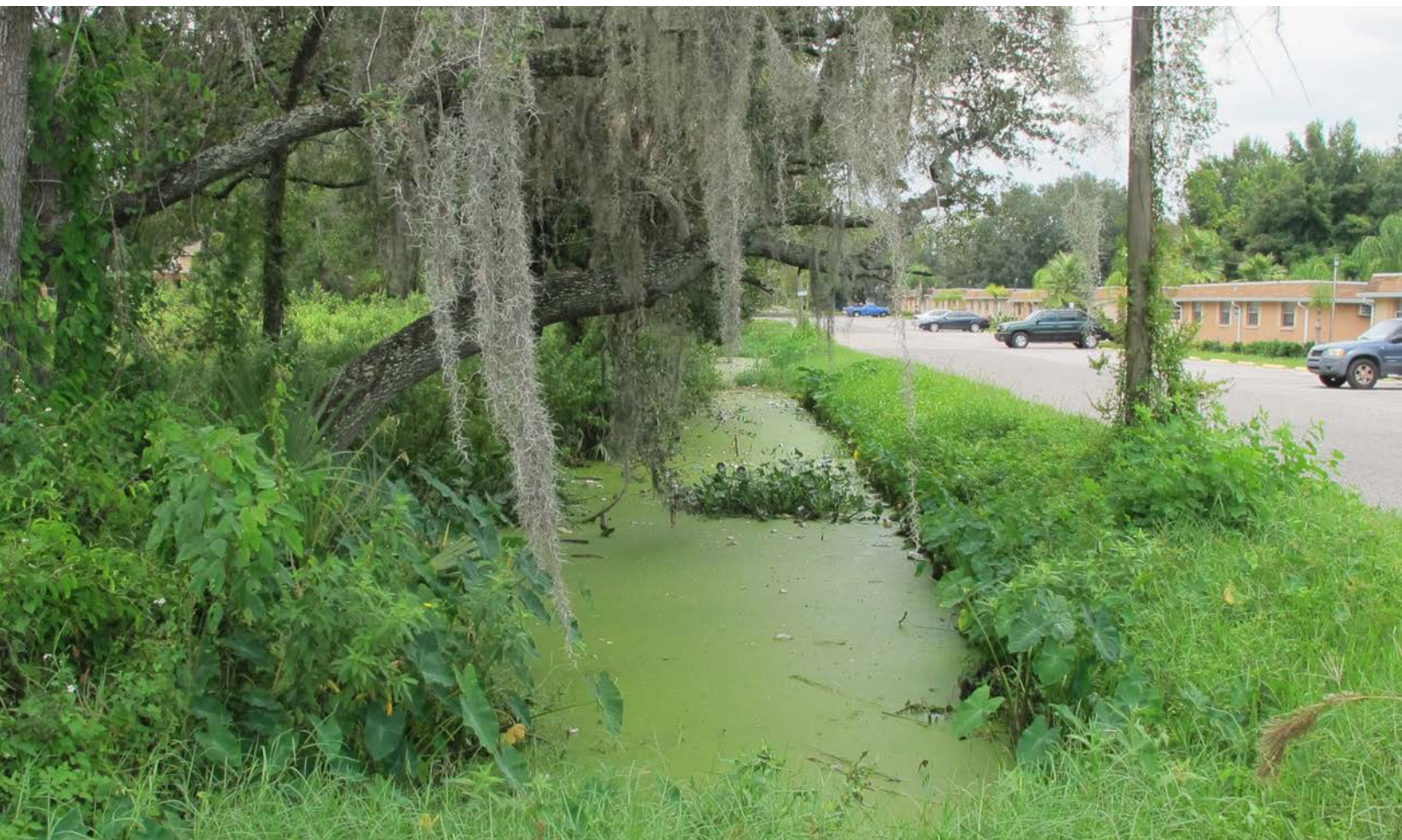
Drainage ditch next to a road with no sidewalk
