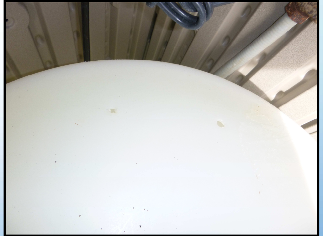
Holes in phosphate day tank
